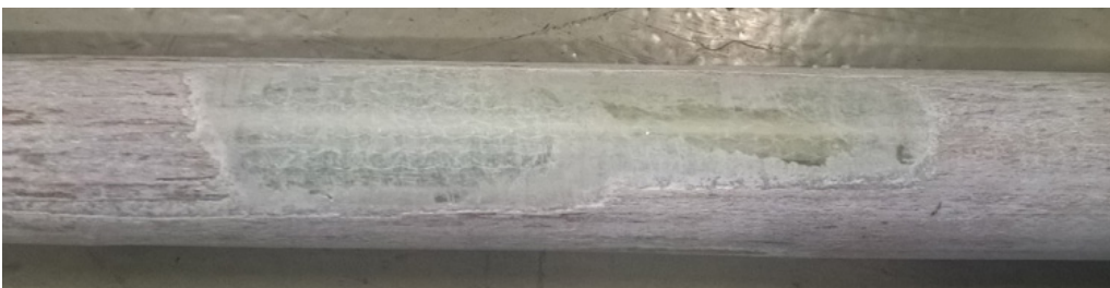
Figure 85 - Bar 6: Abrasive wear top left
