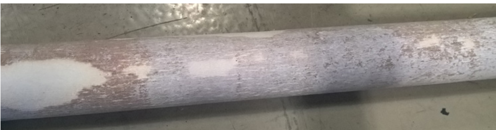
Figure 69 - Bar 2: abrasive wear
