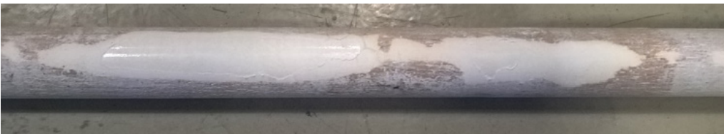
Figure 67 - Bar 2: abrasive wear
