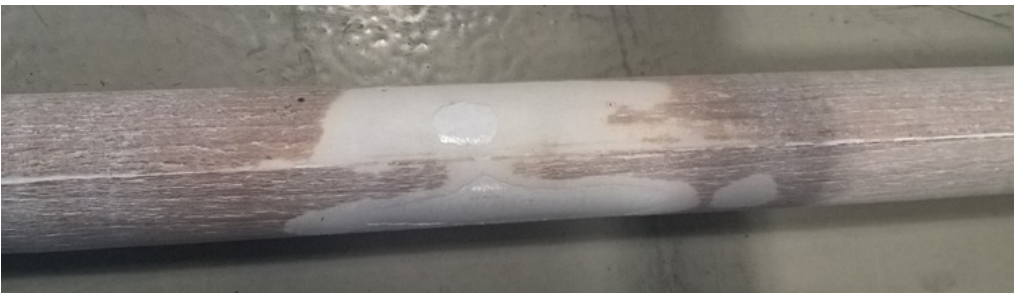
Figure 68 - Bar 2: abrasive wear
